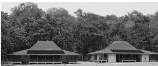
Figure 8. 2x36x300 W<sub>p</sub> distributed on Flora A (left) and on Flora B (right)
