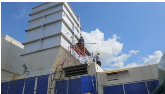
Figure 4. Installing sampling holes
