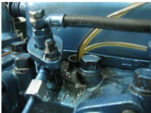
Gambar 2. Instalasi pressure transducer .
