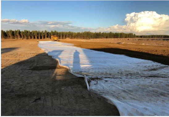
Figure 1. Installation of geotextile underneath new switchyard during construction
